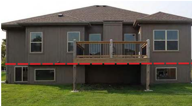
DAYLIGHT FOUNDATION EXAMPLE
