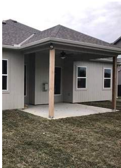
COVERED ROOF OVER PATIO
