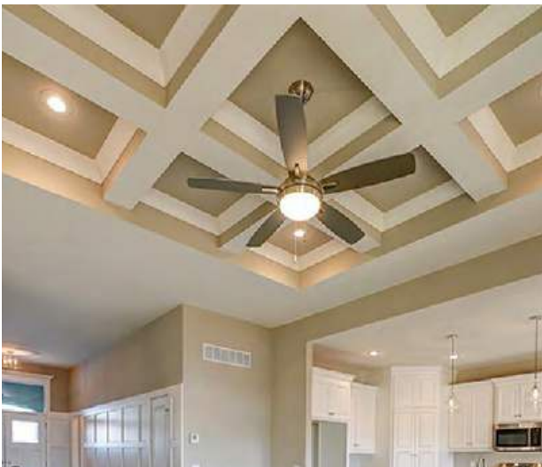
COFFERED WITH COVE INSET
