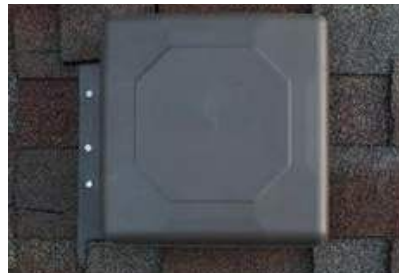
ROOF VENTS up close
