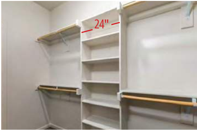
24" STACK IN WALK-IN CLOSETS
