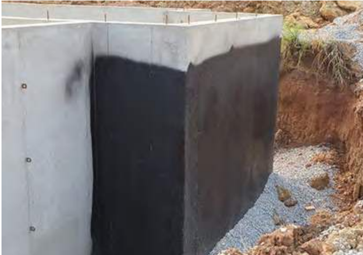
EXAMPLE OF SPRAY ON APPLICATION
