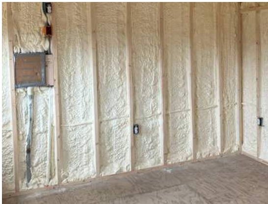
Spray foam insulation in walls
