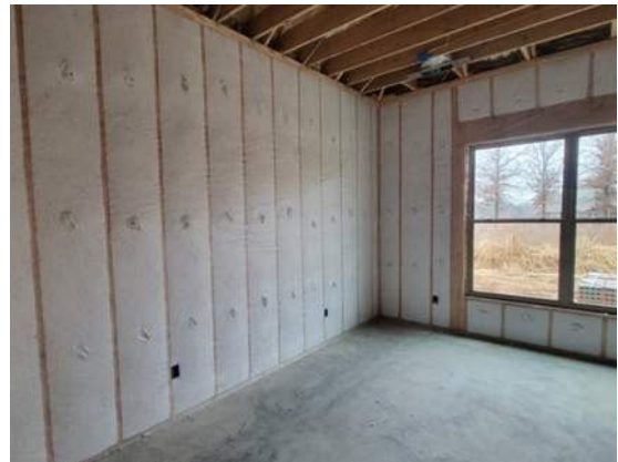
Blown-in-Blanket System insulation in walls
