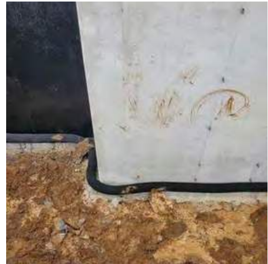
EXAMPLE OF DRAIN TILE (drain tile installed prior to gravel install)
