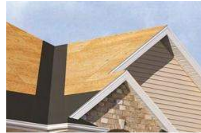
ICE & WATER SHIELD Installed on eaves & valleys
