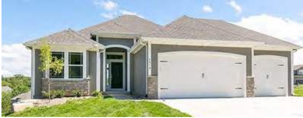
GUTTERS IN WHITE
