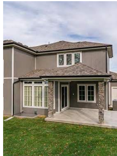
COVERED ROOF OVER PATIO
